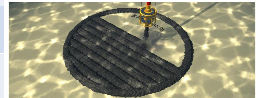
Figure 4-1, Filter layer installation
